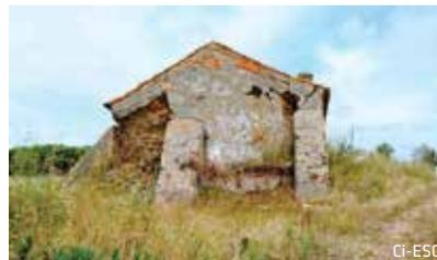
**Fig. 59.** Três contrafortes Three buttresses
