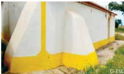
**Fig. 74 .** Contrafortes Buttresses
