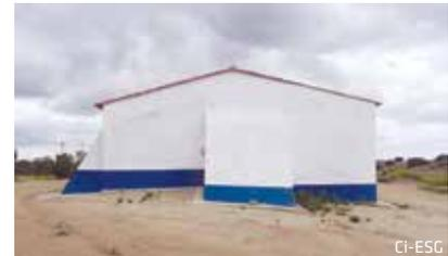
**Fig. 80** . Contrafortes Buttresses
