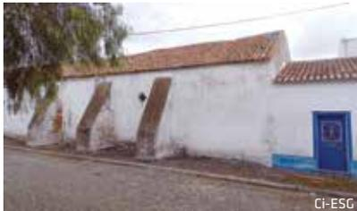
**Fig. 78** . Contrafortes alinhados Aligned buttresses
