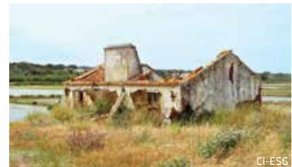
**Fig. 60.** Casa com contrafortes e tirantes House with buttresses and tie-rods
