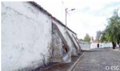
**Fig. 11** . Contrafortes Buttresses
